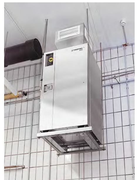
On the exhaust side the larger standing units of the DH series come with a rectangular duct connection for the simply integration in existing ventilation systems. There fan hoses can be optionally connected and upon request we can also realize individual special constructions such as ventilation shrouds.
